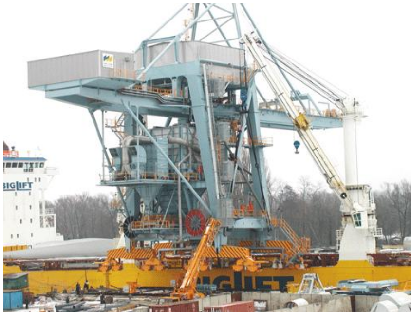
Dust collector for bulk cargo loading in the port of Fremantle
